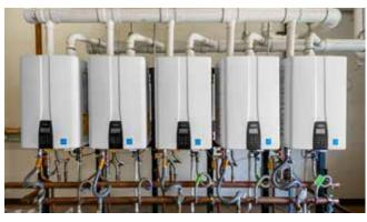
Five NPE-2 Tankless Water Heaters were installed with the Ready-Link Manifold System.
