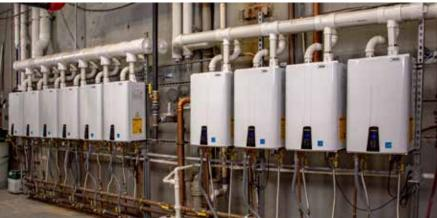
10 NPE tankless water heaters replaced a failing 1.9 million BTU/H boiler to indirect tank system.
