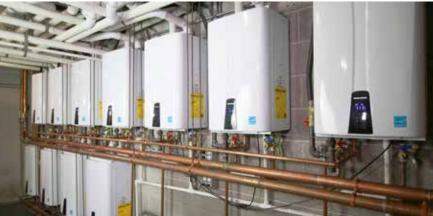
11 cascading Navien NPE-240A units provide endless hot water to the 137-bed facility, complete with commercial kitchen and laundry.
