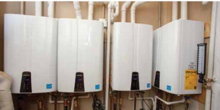
Four Navien NPE-240 units use cascading technology to assure a steady and dependable flow of hot water.
